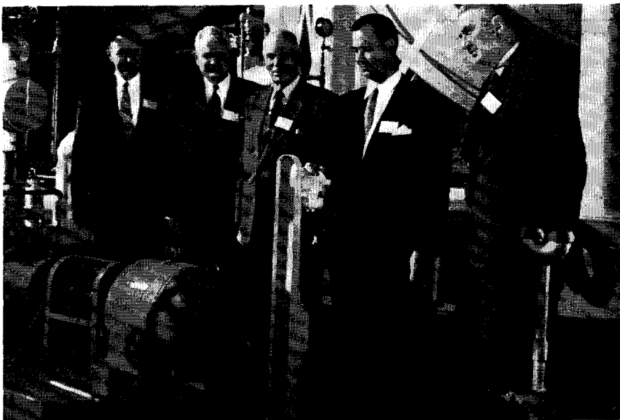
F. D. Kuenzly, plant manager; C. W. Humphreys, vice president; Mayor Petit of Ventura, Calif.; and G. R. Monkhouse, vice president, watch R. C. McCurdy (second from right), president of Shell Chemical, turn the switch putting the new anhydrous ammonia plant into operation
